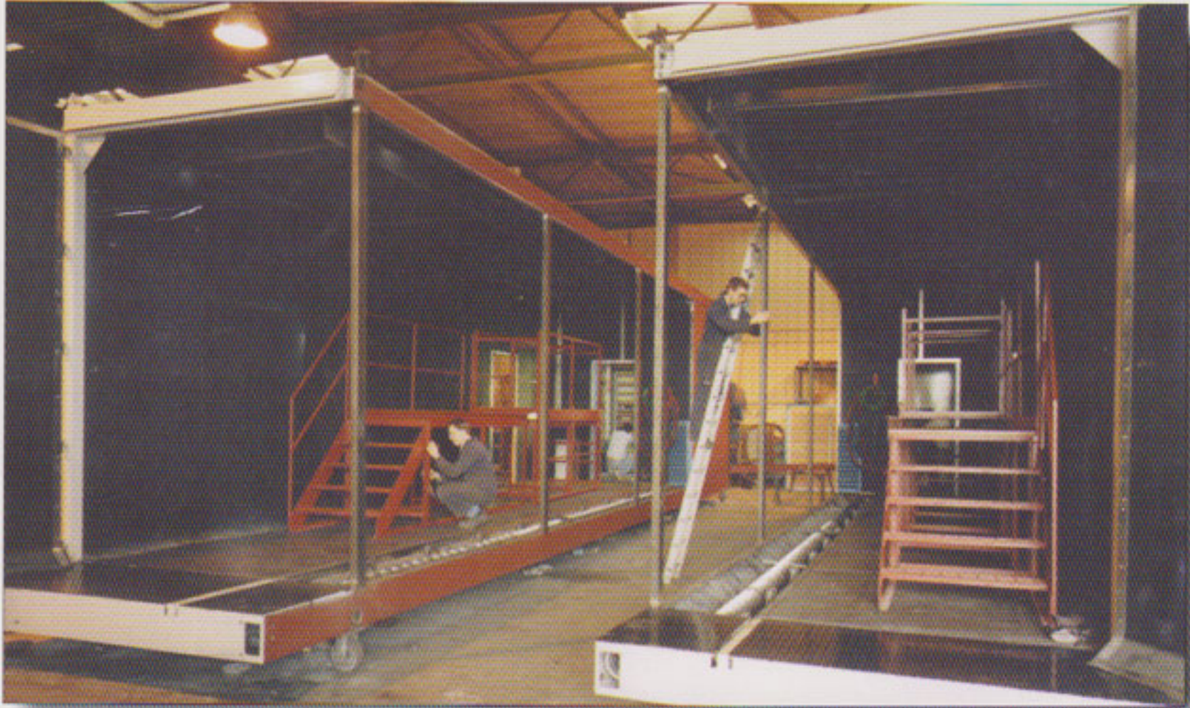
Unit split for transportation - Bahrain Petroleum Company
